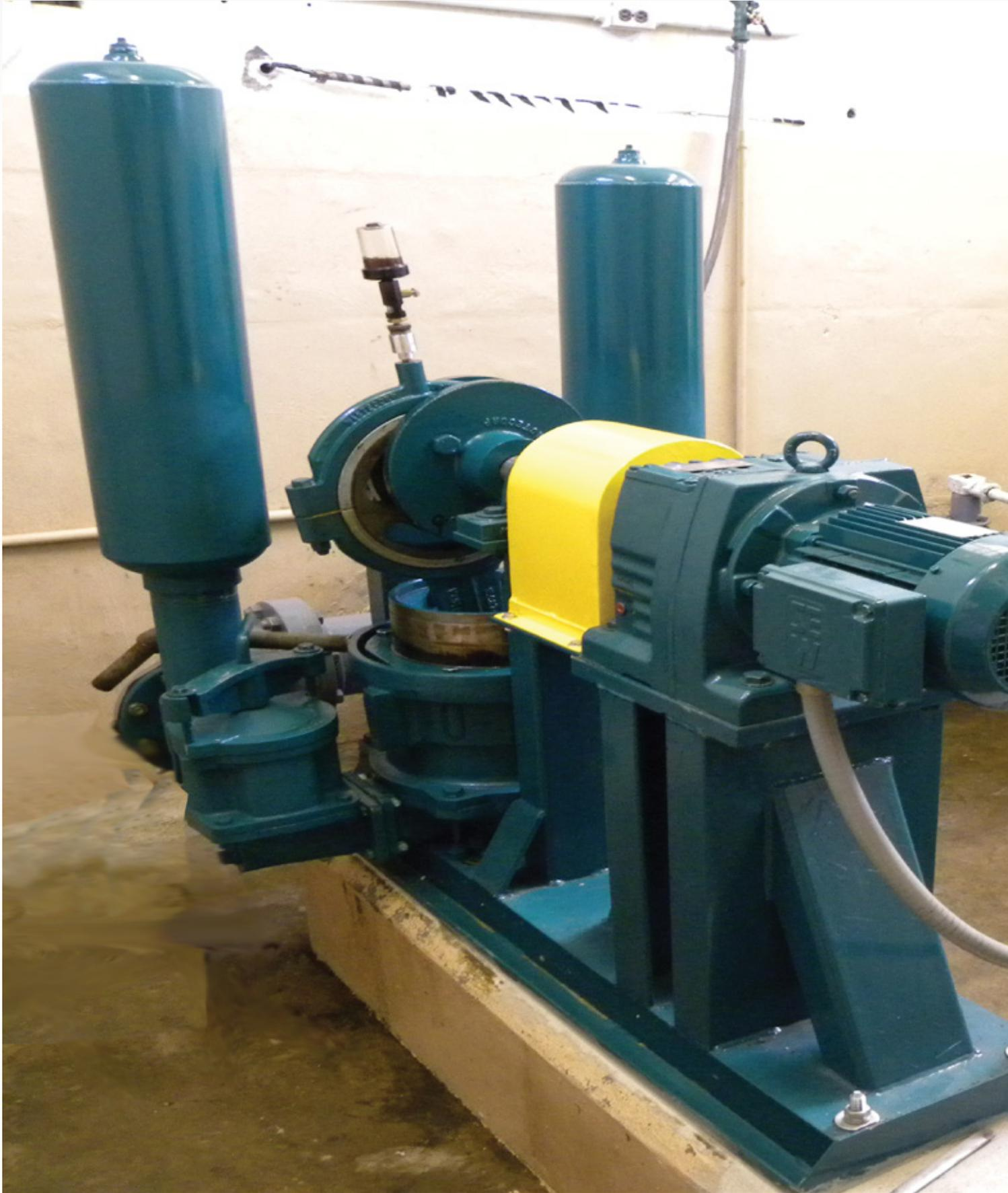
*Wastecorp PE-941 Series at a Palm Beach County, Florida wastewater treatment plant. The PE-941 Series is one of the most popular plunger pump makes to replace rotary lobe and progressive cavity pumps.*
