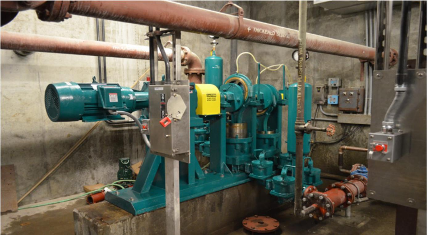
HPE-1142 plunger pump at a Boston, MA water pollution control facility. Pump includes a direct drive motor with a block heater to manage seasonal changes in weather. Higher head application which included dual ball valves for thicker slurry and sludge.
