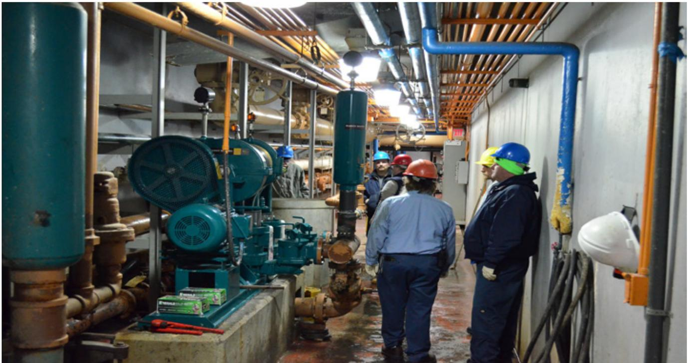
HPE 81W at a New Jersey wastewater treatment plant. The belt driven model has been favored by this facility's operators for decades. When it was time to replace the existing plunger pump the operators opted for the same belt driven design for enhanced pumping productivity.
