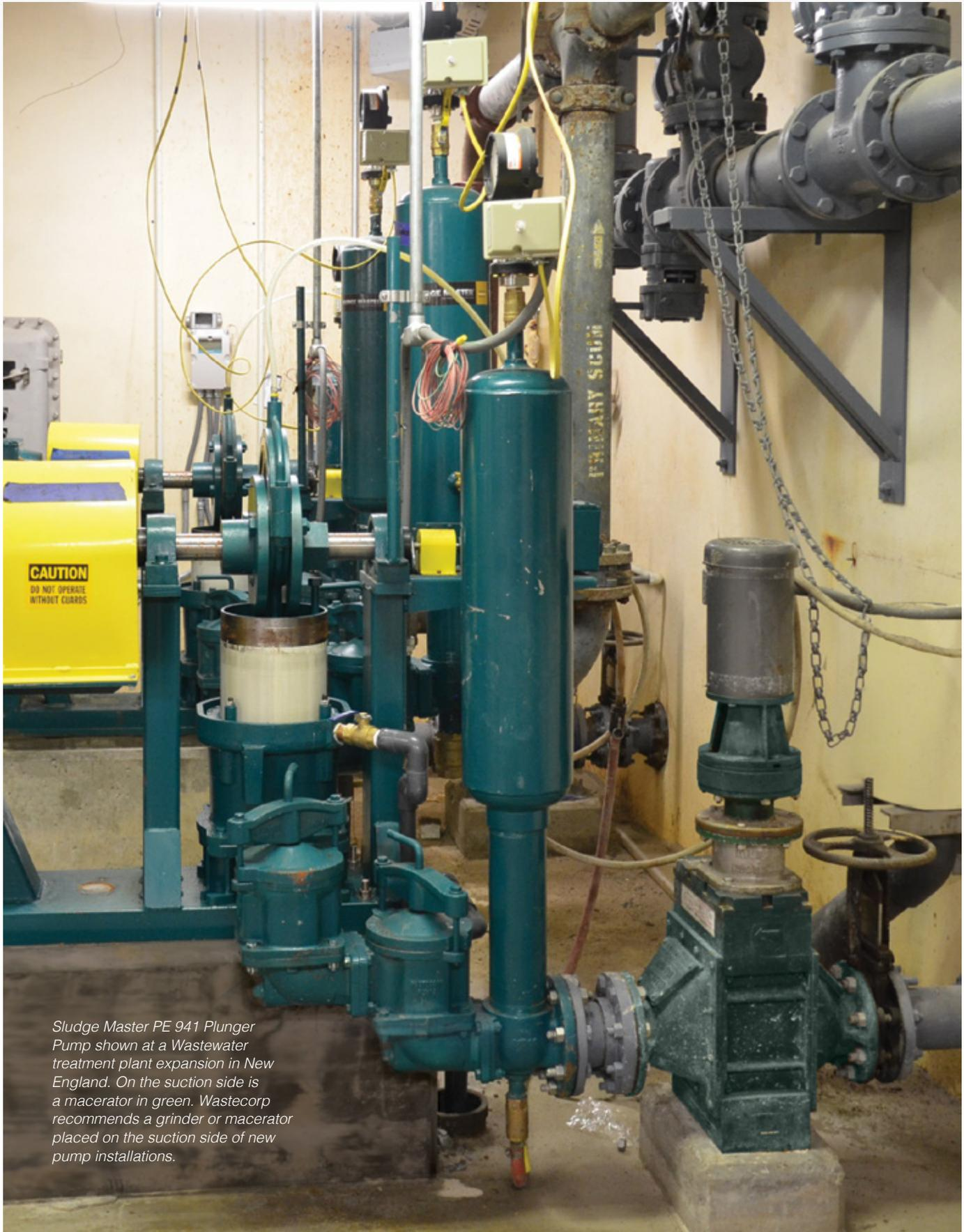
*Sludge Master PE 941 Plunger Pump shown at a Wastewater treatment plant expansion in New England. On the suction side is a macerator in green. Wastecorp recommends a grinder or macerator placed on the suction side of new pump installations.*
