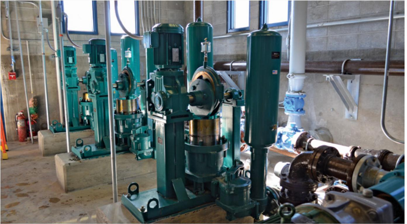
Model PE-9-SS Plunger pump in a Riverside County, California wastewater treatment plant. The facility replaced rotary lobe pumps with next generation plunger pump technology. The space saving design shown reduces the pump footprint by 35%. Application involves pumping thickened fermented sludge from a digester.
