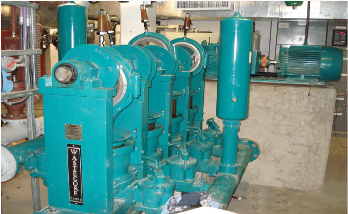
Wastecorp EHPE Series installed at a City of Edmonton, Alberta Canada wastewater treatment facility. Wastecorp installed eight plunger pumps at the facility as part of a multi-year upgrade/expansion.
